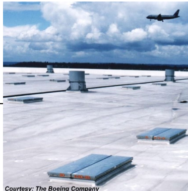
SMOKE & HEAT VENTS (IFC 910.3)
